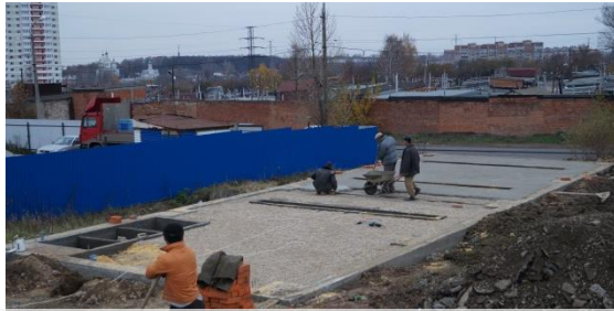
№1. Making a lighter foundation for a small autoshop centre.
