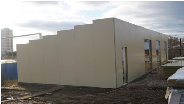
№4. Mounting of both wall and roof composite sandwich panels using screws, fittings and fasteners.
