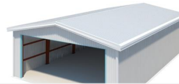
Designing of a wide opening for large vehicles on the endwall sides
